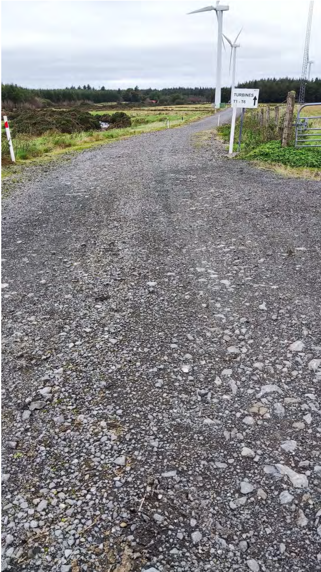
Plate 4-2 Typical existing site road
