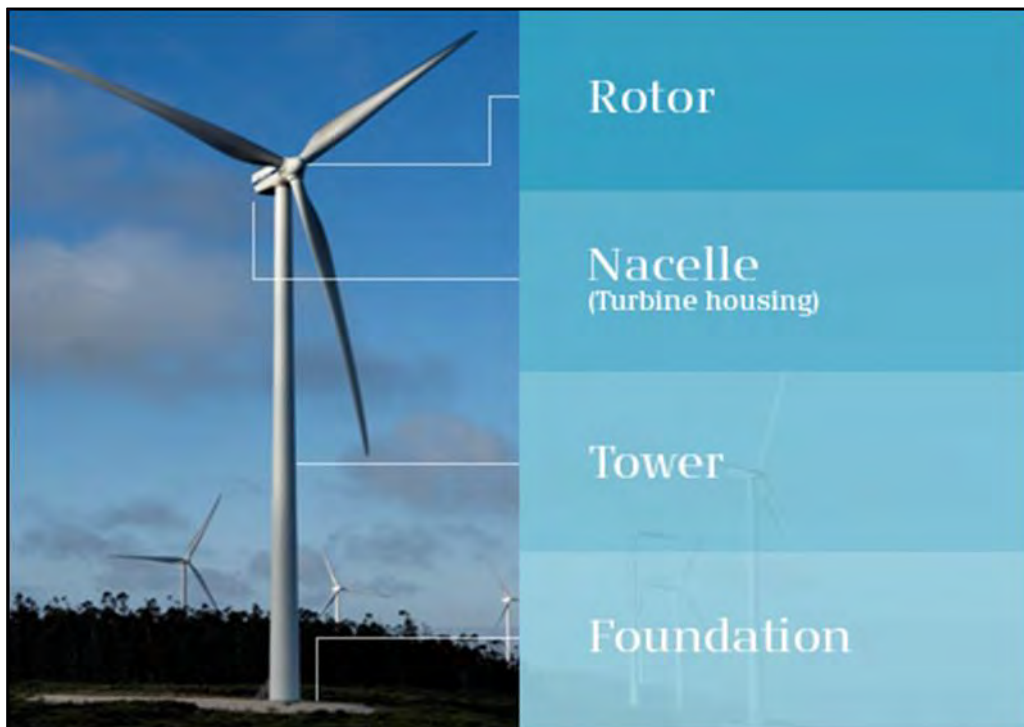
Plate 4-1 Wind turbine components
