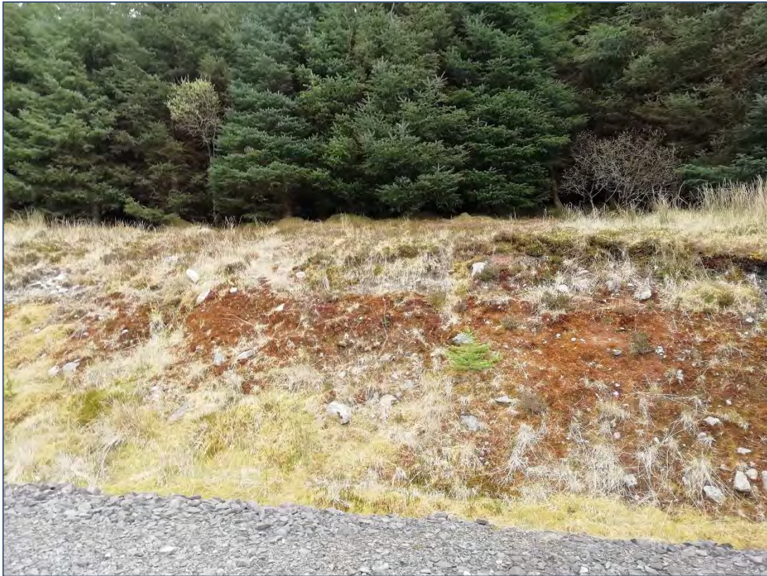
Plate 6-2: Earth banks (BL2) adjacent to T13.
