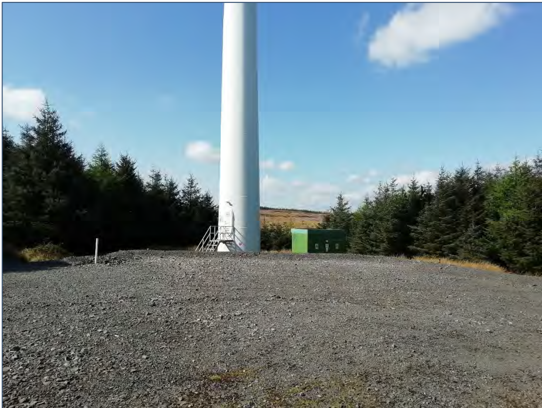
Plate 6-1: Hardstanding area and turbine (BL3)
